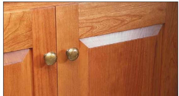
My shop-built cabinets feature 3/8" inset, solid cherry raised panel doors with wide rails. These features weren't available in stock cabinetry.
