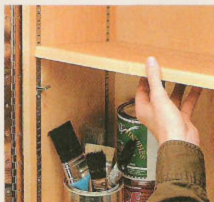
C. Adjustable Shelving. Metal shelf standards allow you to adjust the shelving for your storage needs.
