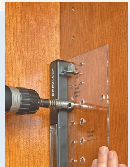
▲ Continuous Drilling. Slip a shelf pin in the indexing hole to keep drilling down the workpiece.
